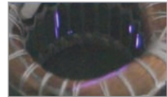
Figure 8: Corona discharge in motor
