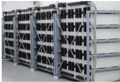
Energy Storage System
