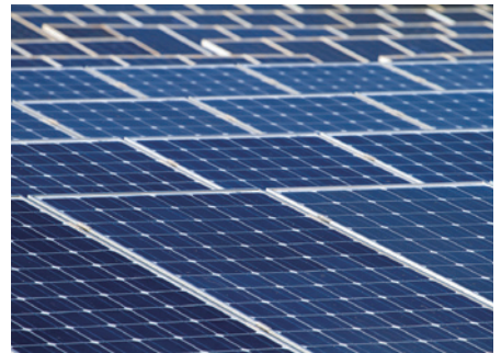
Solar Array Load Testing
